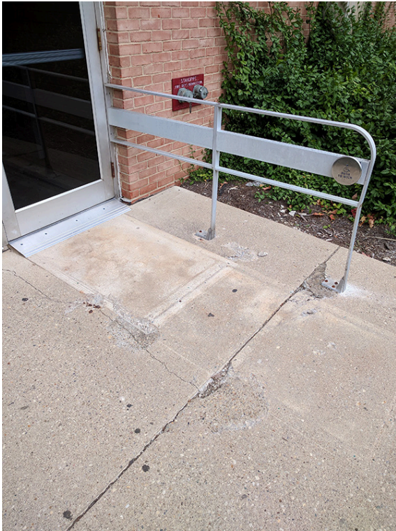
Deterioration of sidewalk at accessible building entrance.
