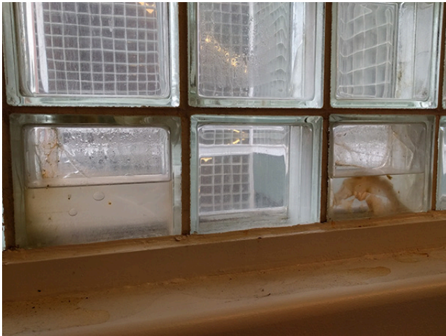
Water infiltration in glass block, Medical Sciences.
