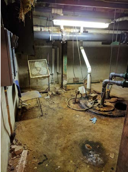
Deteriorated sump pump and mechanical area at swimming pool.
