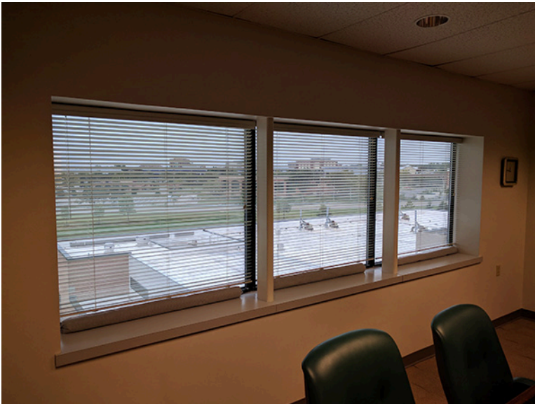
Absorbent socks on the window sills to deal with repetitive leaks, Russ Engineering.
