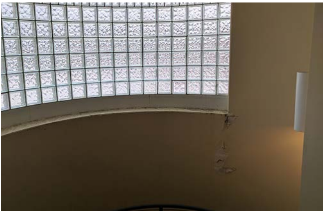
Water damage in Russ Engineering stair tower.
