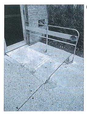
Deterioration of sidewalk at accessible building entrance.
