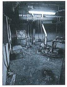
Deteriorated sump pump and mechanical area at swimming pool.
